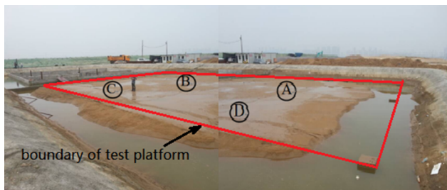
Fig. 11. Sand foundation after sand filling.
